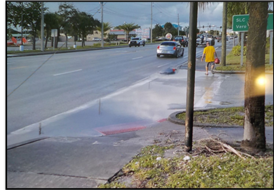
SR 5/US 1 at Tennessee Avenue Pre-Construction
