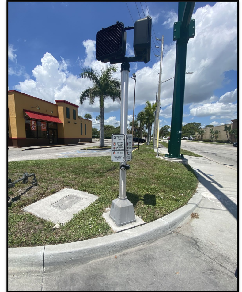
Pedestrian signal at the SR 5/US 1 and Ohio Avenue Intersection Pre-Construction
