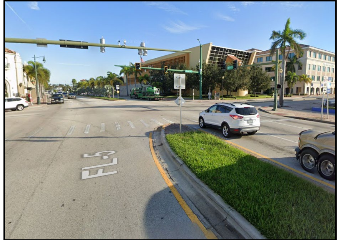
SR 5/US 1 at SR 68/Orange Avenue Pre-Construction
